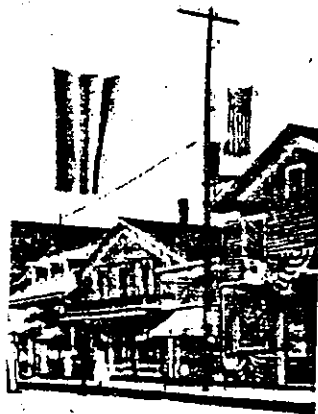
RECORD OFFICE AT RIGHT (East Side of Center Street)
